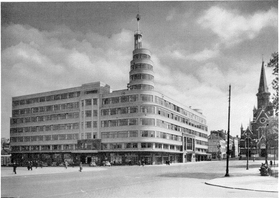
Fig. 1—Broadcasting House of Institut National Belge de Radiodiffusion in Brussels.
